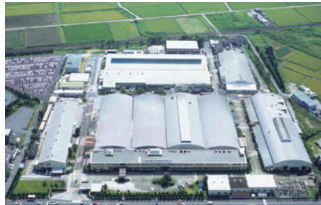
MITSUBISHI MATERIALS AKASHI PLANT (JAPAN)
