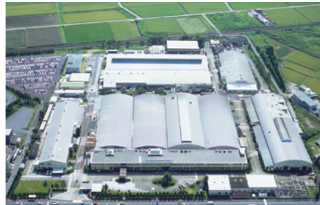
MITSUBISHI MATERIALS AKASHI PLANT (JAPAN)
