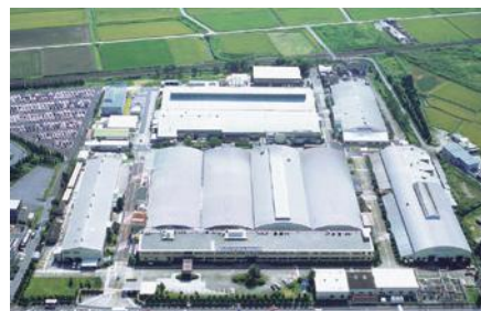
MITSUBISHI MATERIALS AKASHI PLANT (JAPAN)
