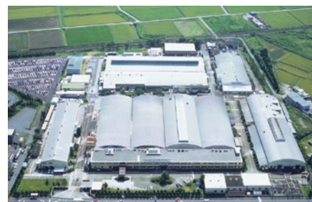
MITSUBISHI MATERIALS AKASHI PLANT (JAPAN)
