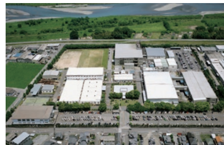
MITSUBISHI MATERIALS GIFU PLANT (JAPAN)
